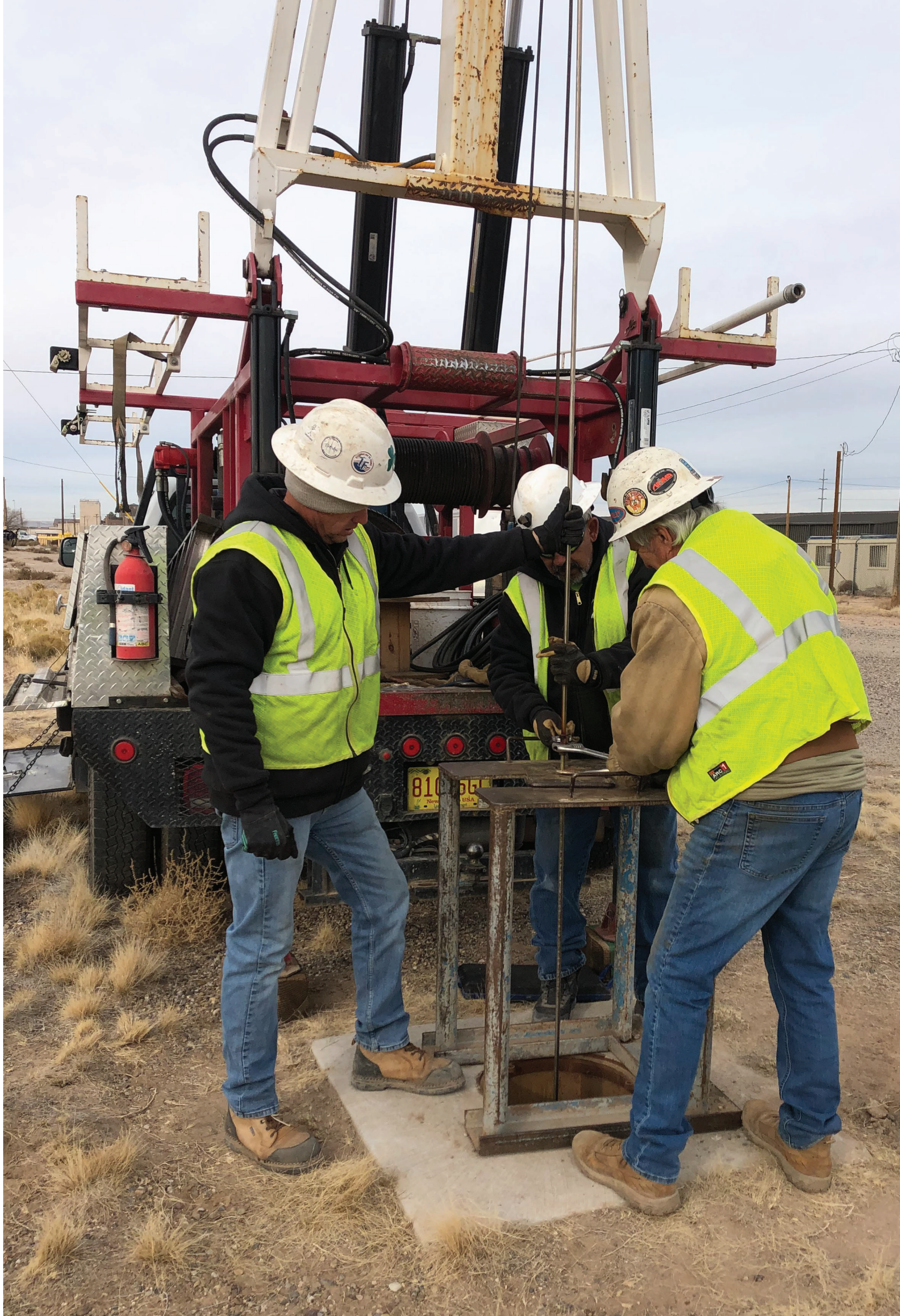
Removing the failed pump in KAFB-106024
