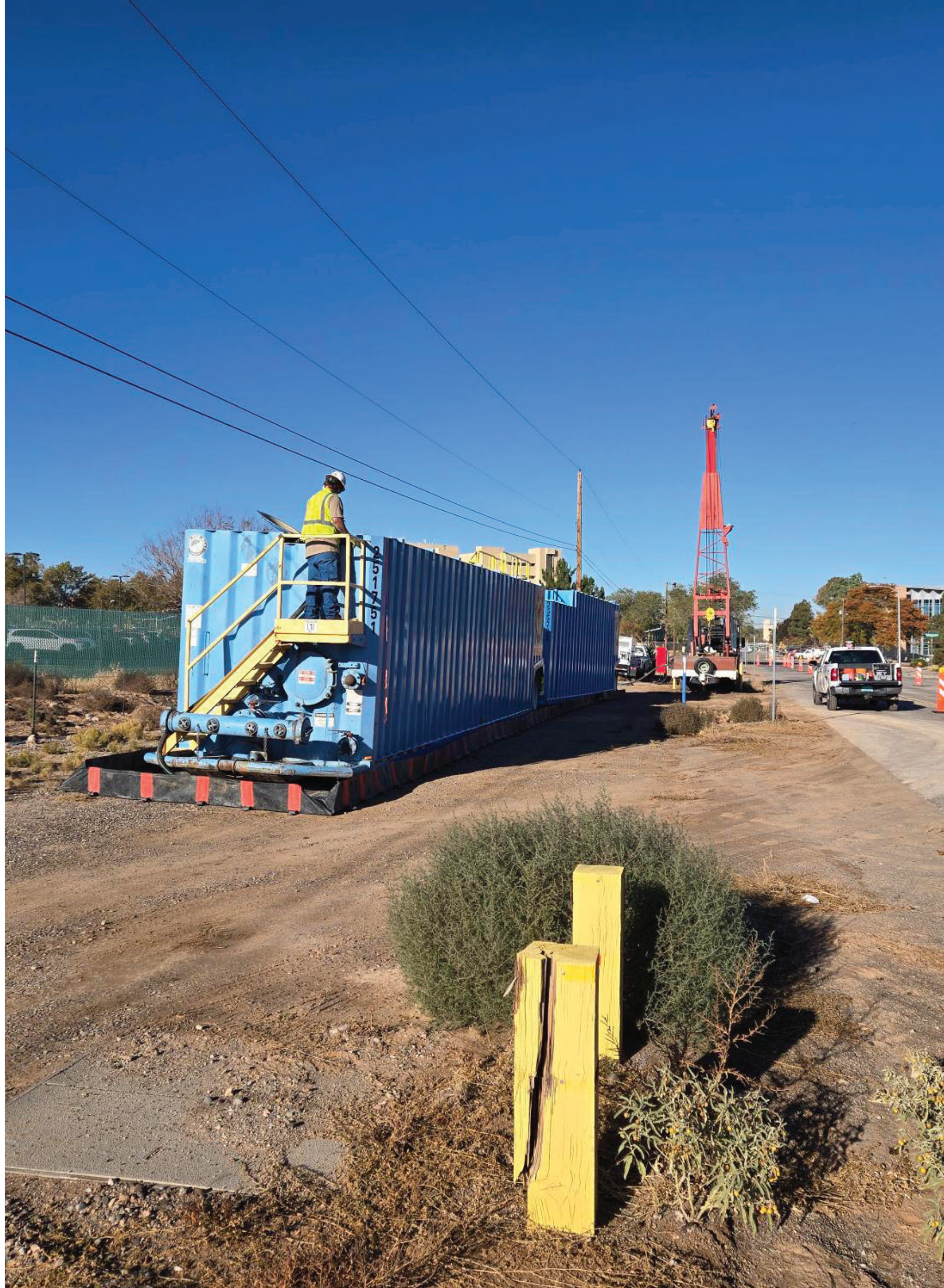
Extraction well KAFB-106239 rehabilitation
